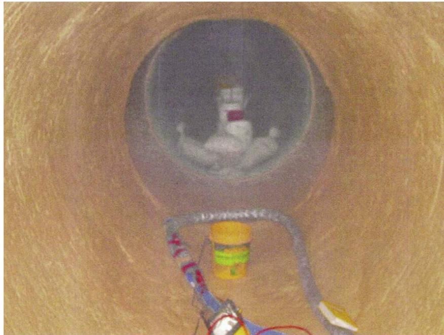
Fig. 6: Robotic sprayed-in-place pipelining
